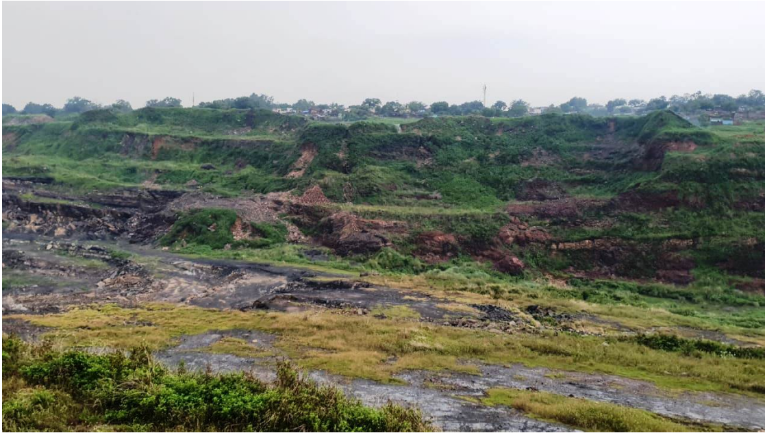
Figure 19: Subsidence area in Bagdigi Mines
